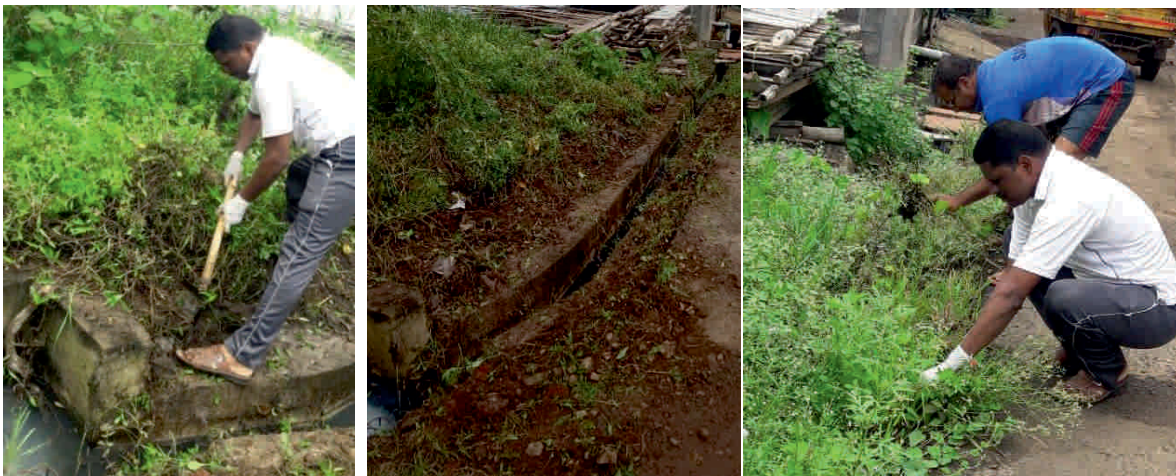
After and Over Cleaning Efforts
