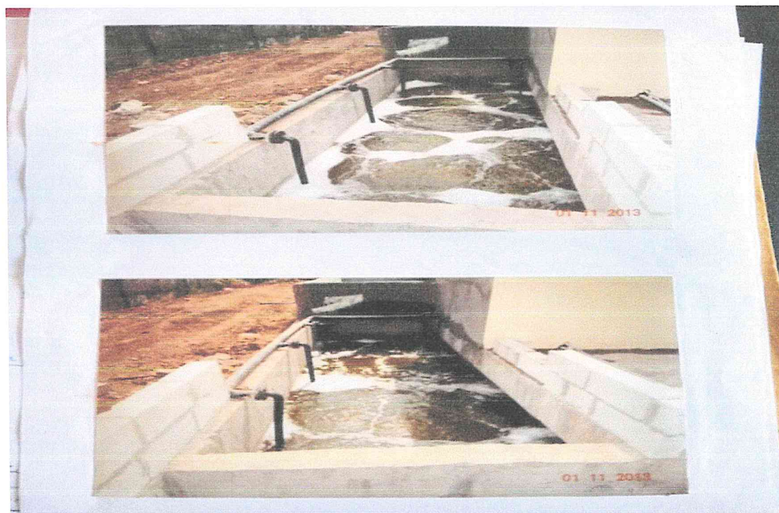
Sewage treatment plant
